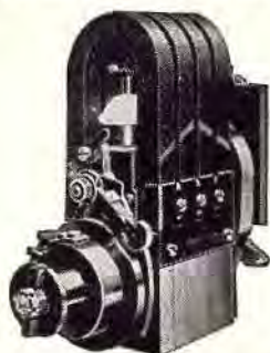
Diagram E, showing impulse starter mounted on the K. W. high-tension magneto.
