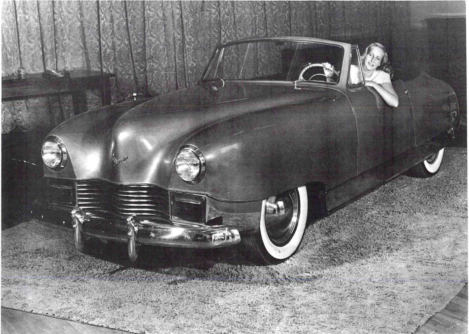
DARRIN CAR (1945) WITH WIFE AT THE WHEEL. THIS CAR HAD FULL TILT FORWARD HOOD AND FENDER ASSEMBLY, AND SPRING LOADED LICENSE PLATE FRAME TO HIDE GAS CAP.
